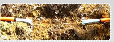
Peal off outer sheath of MD after cutting off the impaired part
