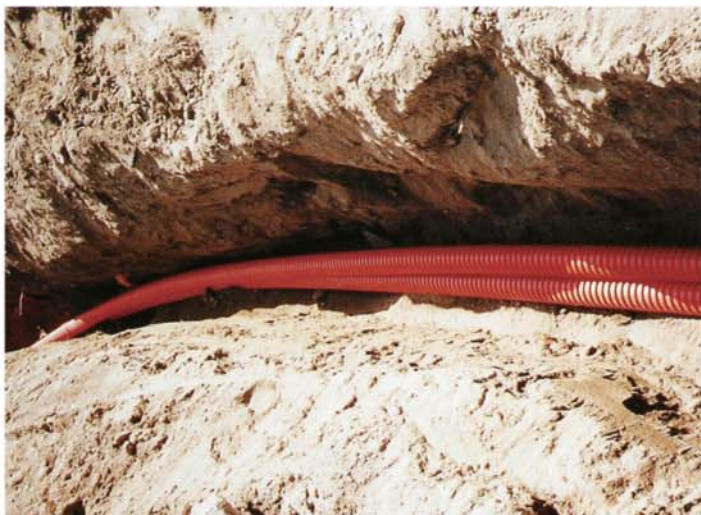
▲ Roll mounted COD releases and straightens easily for installation
