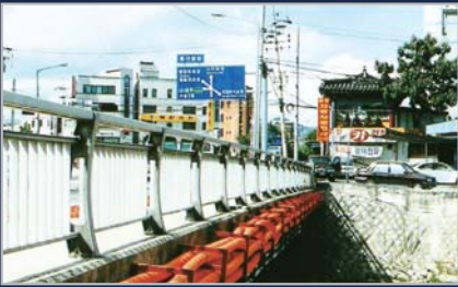
Installed along with bridge
