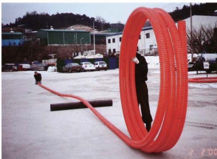
▲ COD by-passes hurdles owing to its flexibility
