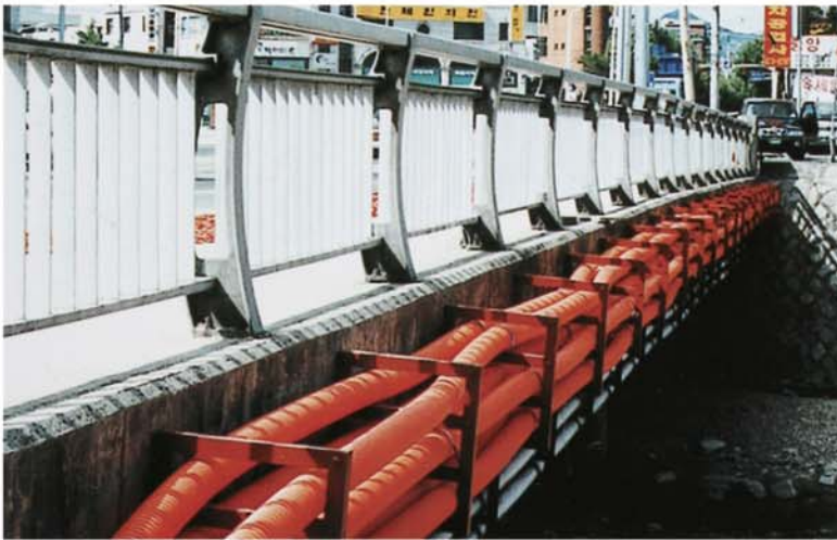
▲ Installation along with bridge: COD with UV protection.
