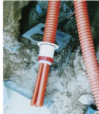
▲ Ready for connection manhole.
