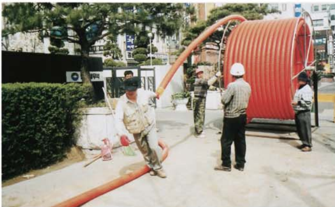
▲ Easy releasing COD from spool.
