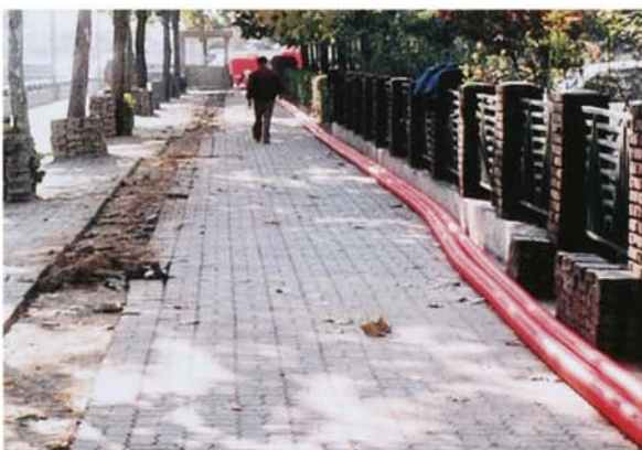
▲ Temporary COD laying along walkway.
